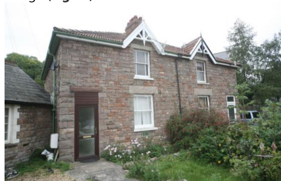
Fig.64 The Quarries feature squared stone
