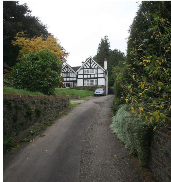
Fig.106 St Govans set back off the roadside in its own private grounds
