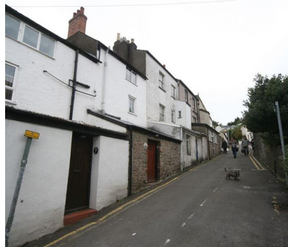
Fig.91 The rear elevations of Mount Pleasant terrace on Steep Street – the main entrance to these houses is from Steep Street despite their original architectural orientation to the south-east
