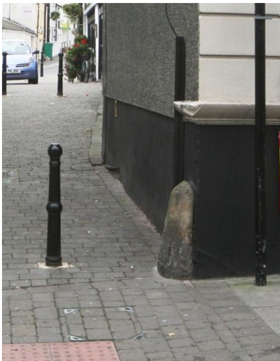
Fig.83 Stone buffers featured on buildings were used to protect buildings from being struck by wagon wheel hubs.
