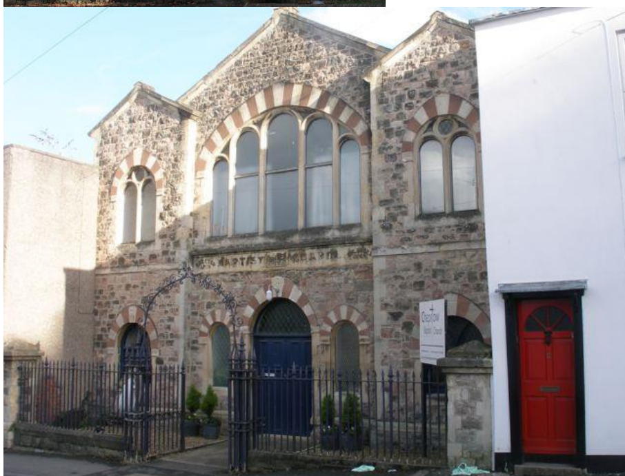
Fig.140 The Baptist Church (1869). A freer interpretation of pre classical architecture, with hints of the Venetian Romanesque.
