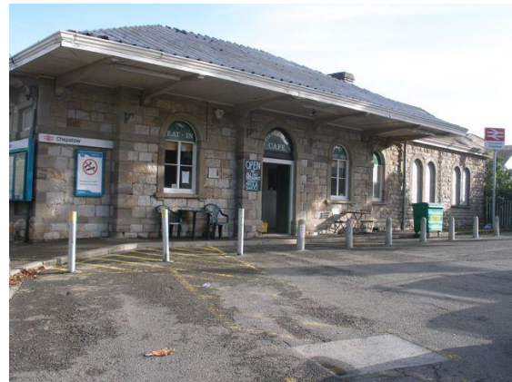
Fig.143 The Railway Station, built to the designs from Brunel's office. The Italianate style is used for its simplicity and good proportions. The roof is a replacement.
