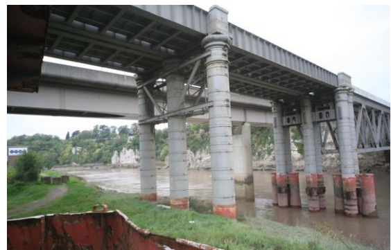
Fig.58 Brunel's railway bridge
