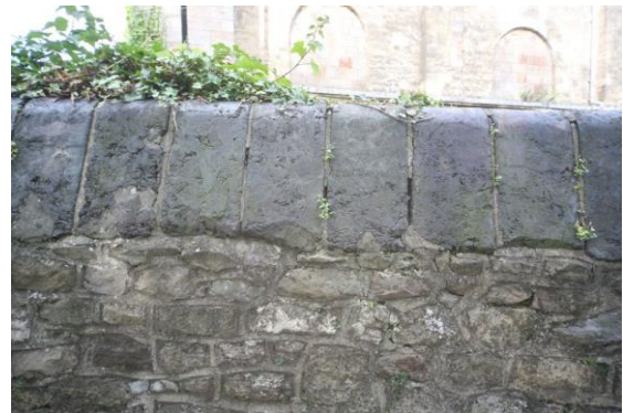
Fig.34 Slag blocks are a feature of special note
