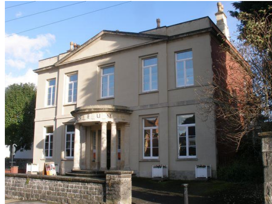
Fig.132 Gwy House, the Chepstow Museum; a refined Palladian style house with correct Tuscan columns supporting a semi circular portico.
