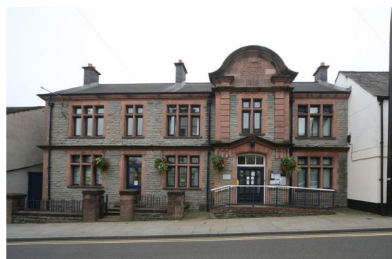
Fig.78 The rock-faced stone Police Station (1912)
