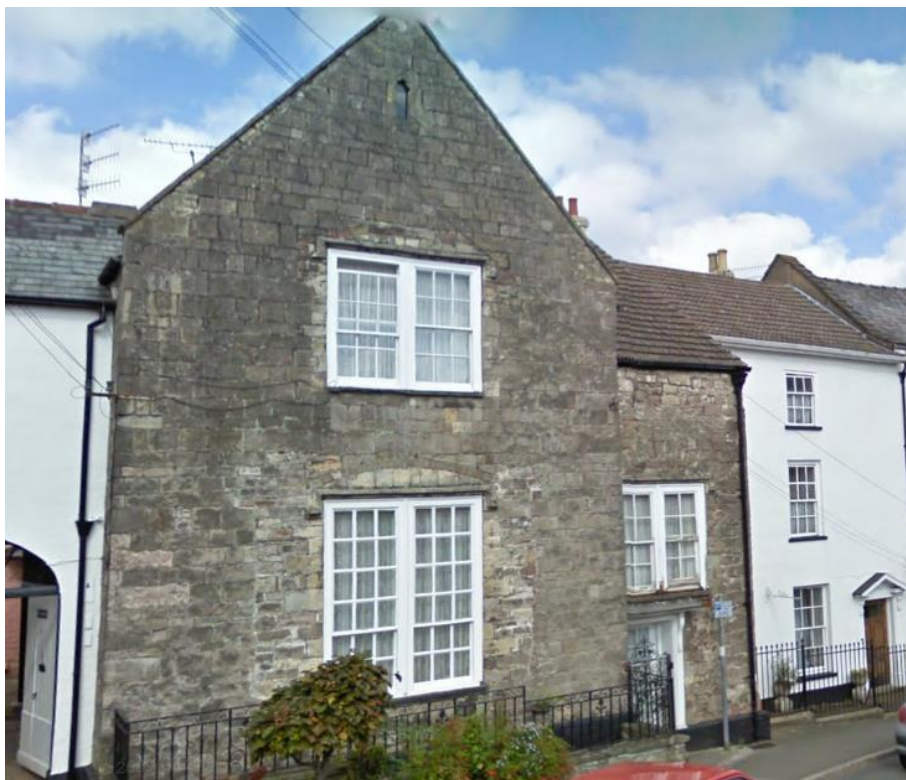
Fig.119 St Ann's. The original medieval gable and layout remains, although the windows are later alterations.
