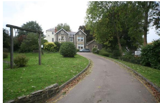
Fig.107 Boverton House, a large detached property. Its large grounds reflective of the character of the area
