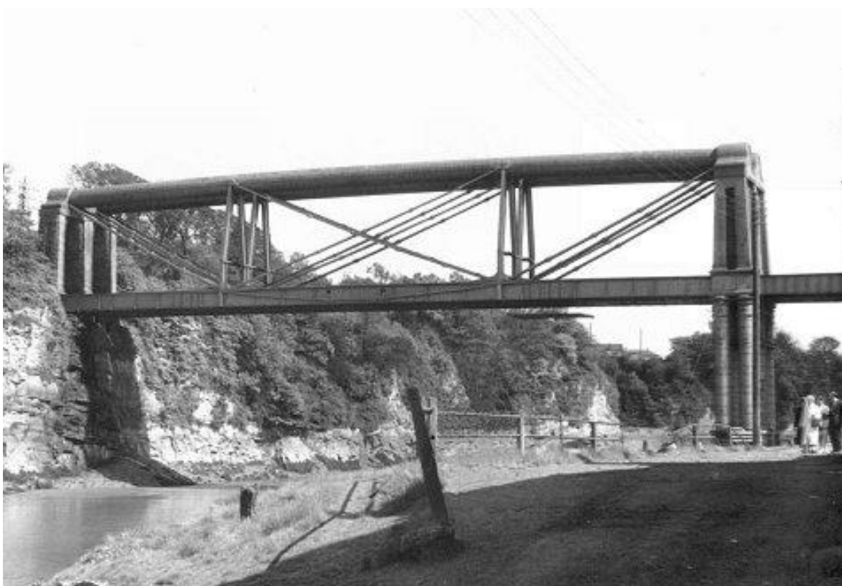
Fig.11 Brunel's railway bridge over the River Wye before its replacement in 1962
