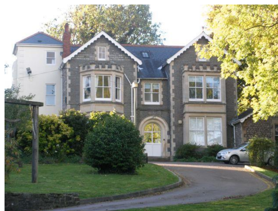
Fig.142 Gothic Revival house. This flexible style could be applied to most building types; here battlements, gables and mullions are applied to a large detached house.
