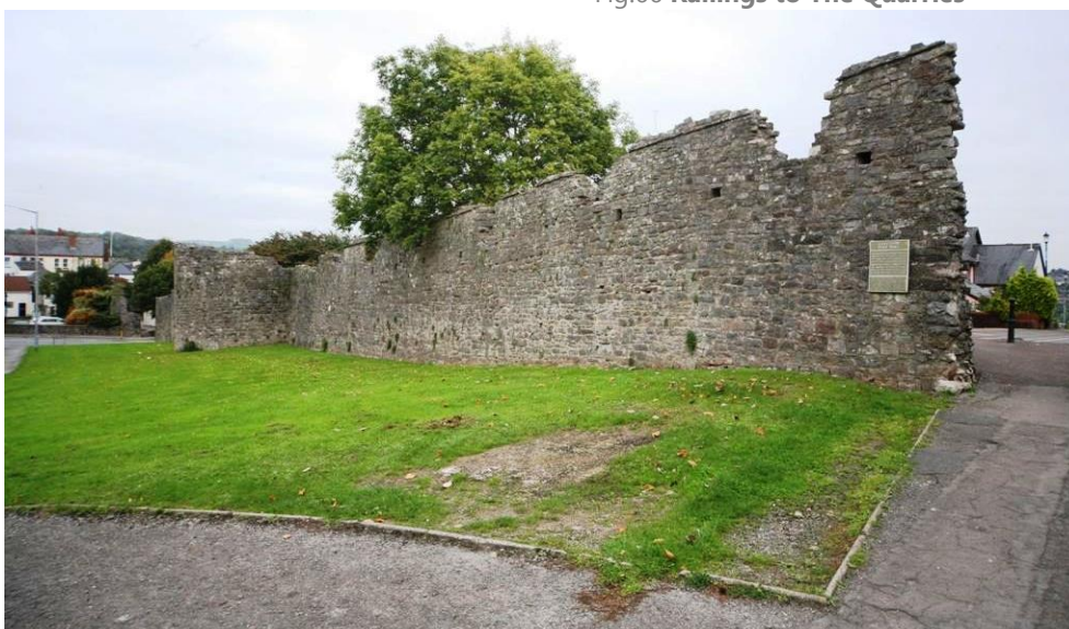
Fig.65 The Port Wall is a Scheduled Ancient Monument of national significance
