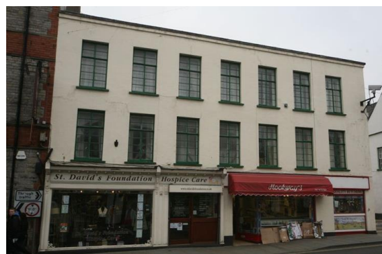
Fig.76 Metal casement windows are a feature of Nos. 18-19 Moor Street
