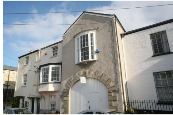
Fig.158 A typical group of rendered houses along Lower Church Street, note the incised render to the right-hand property
