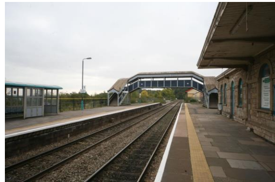
Fig.62 The 1892 cast iron footbridge
