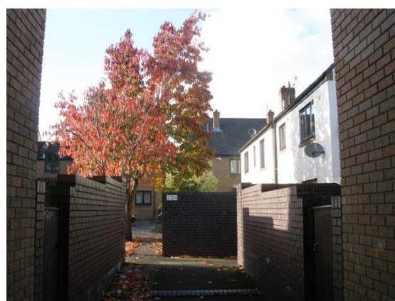
Fig.153 Hollins Court, a successful infill scheme which received a housing award in 1985, creates an intimate network of lanes and 'places'.
