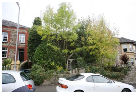
Fig.96 Rosedale, part of a significant group but almost entirely encased in vegetation
