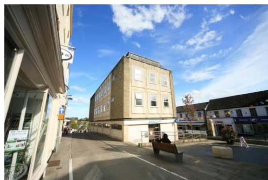
Fig.20 The 1960s Barclays Bank introduces a bold 20th century dimension to the High Street
