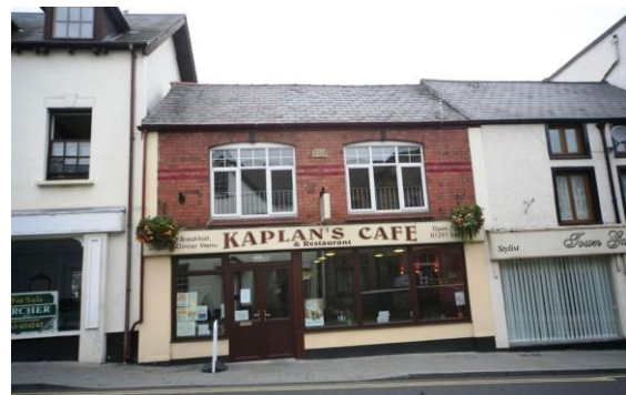
Fig.160 Natural slate is a typical roofing material seen in the conservation area
