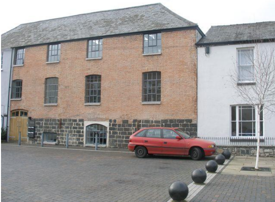
Fig.138 Warehouse adjacent to Wye House. The plinth is constructed of furnace slag blocks.
