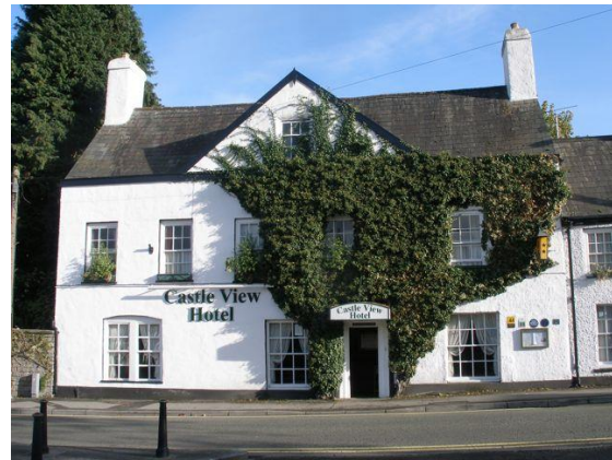
Fig.127 Castle View Hotel: 18 th century with characteristic Chepstow gable, plus Georgian sashes.
