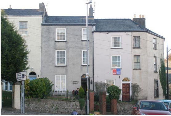
Fig.137 Mount Pleasant, another of the terraces of Chepstow, this time from the 1830s, but still adhering to Georgian principles.
