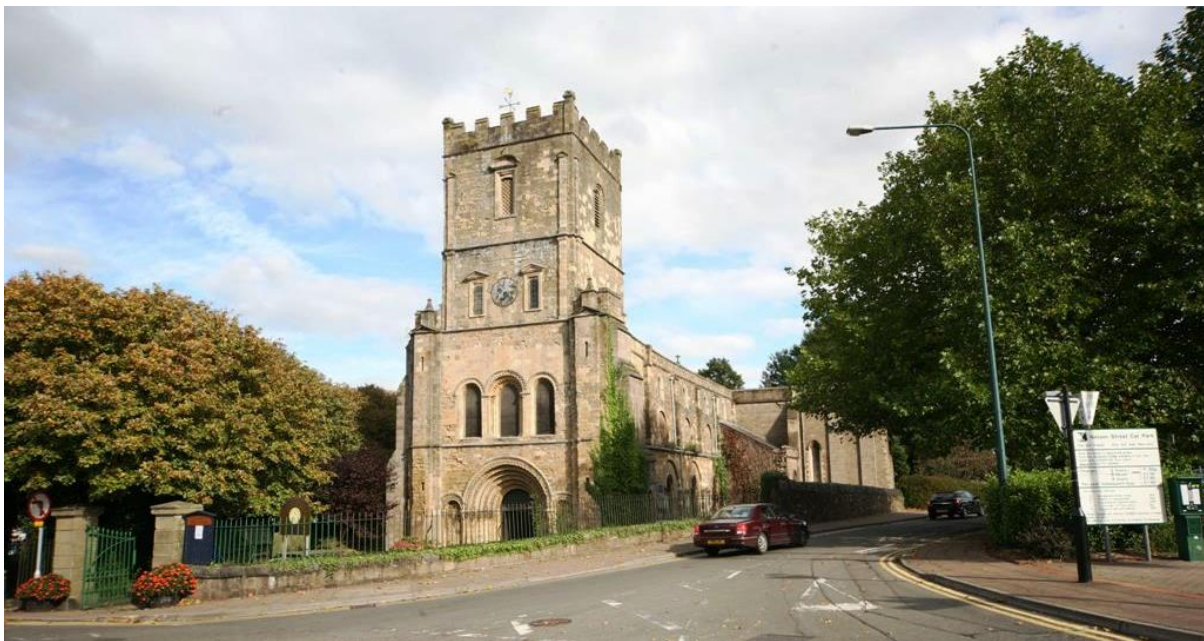
Fig.117 St Mary's Church from the south-west. The Norman and 18 th century stages of the tower are clearly visible. The Victorian south transept can be seen to the right.
