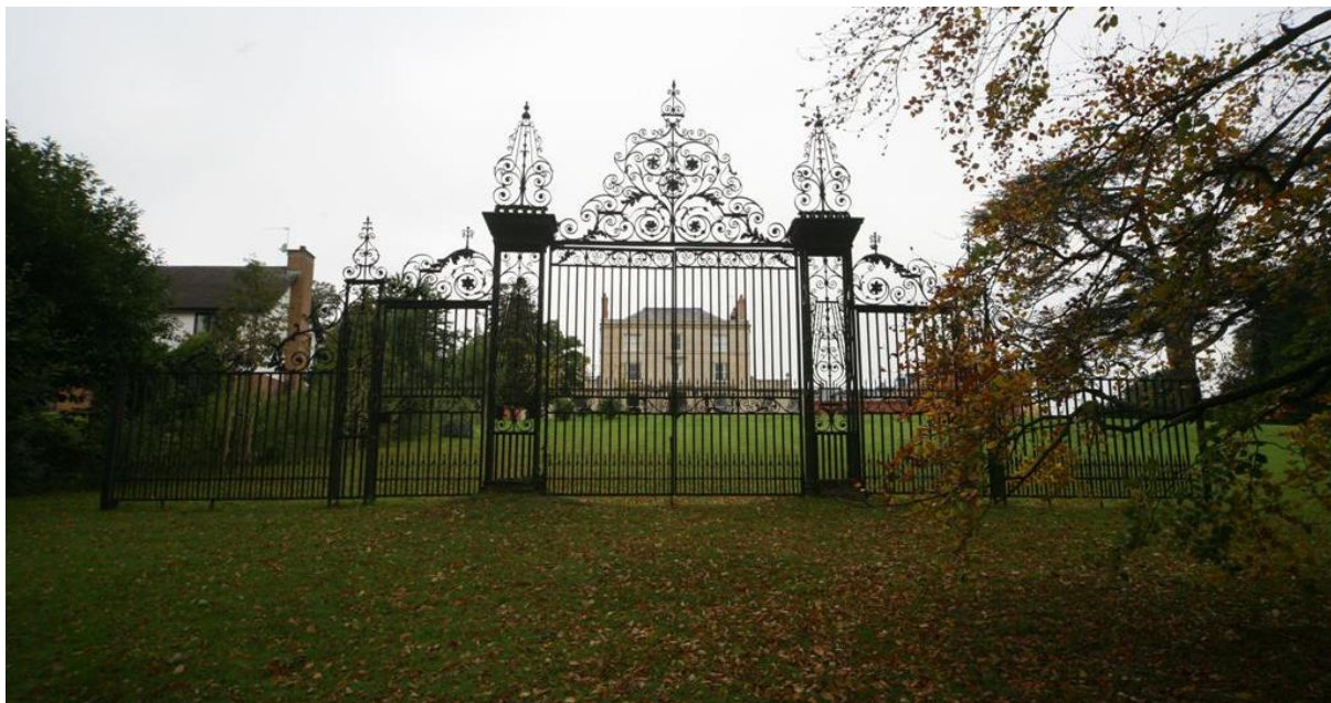
Fig.89 The well executed and highly decorated Grade II listed gates to The Mount
