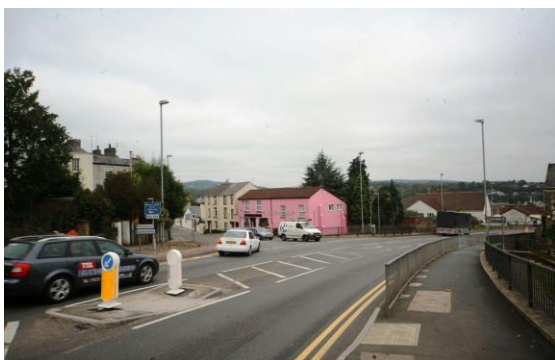
Fig.101 No. 3 Hardwick Terrace (mostly given its chosen colour scheme) terminates views north-east along the A48
