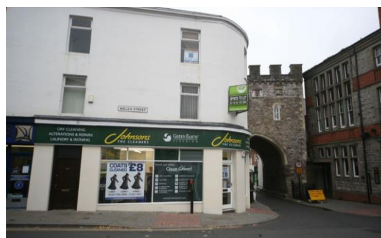
Fig.71 Distinctive curved corner buildings address the junction of Welsh Street and Moor Street
