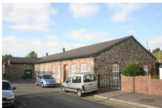
Fig.157 Use of rubblestone with red brick dressings on the Drill Hall
