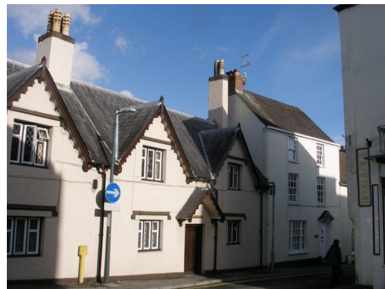
Fig.123 Sir Walter Montague Almshouses, founded in 1614, with a characteristic low roofline and multiple gables, altered in the 19 th century.
