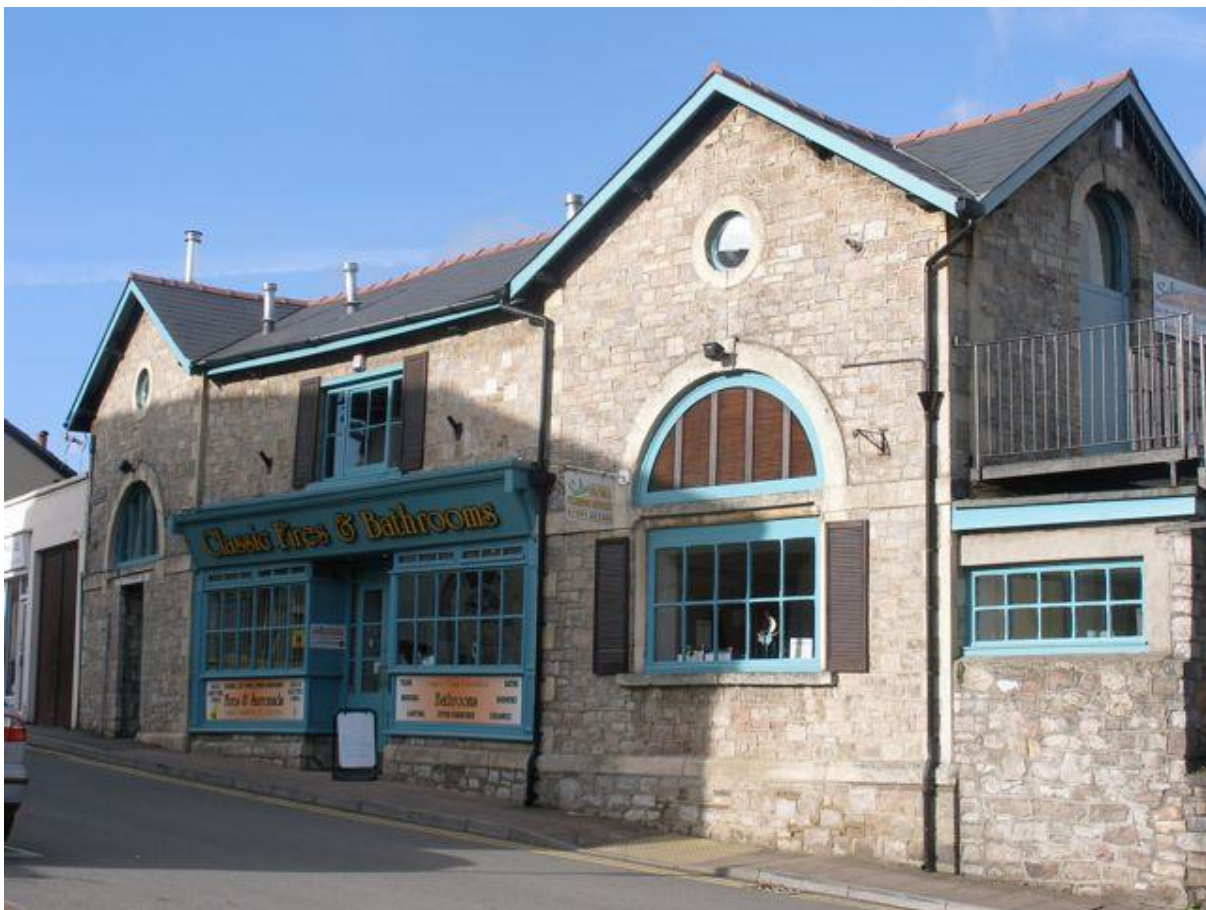
Fig.144 Shop, Station Road. Italianate design principles enhance this functional mid-19 th century commercial building.
