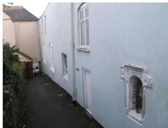
Fig.120 Late medieval window. Some medieval features survive behind 18 th century refronting. This is to the rear of Manor House, Beaufort Square.
