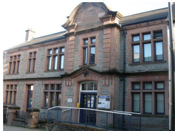
Fig.149 The Police Station, a sober and solid Edwardian building, but also effective in its use of Freestyle design.
