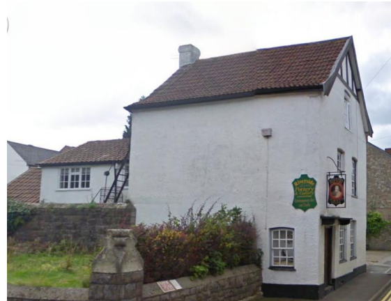
Fig.121 Cromwell House. A rare 16 th century house with its gable to the street. Oliver Cromwell stayed here during the Civil War.
