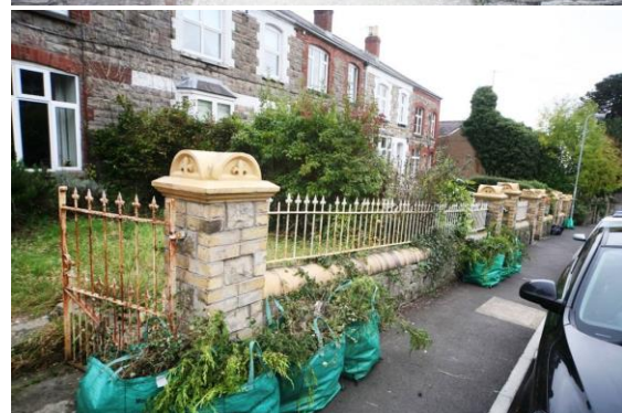
Fig.102 Examples of the good survival of historic ironwork in the character area
